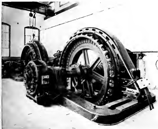
FIG. 5.—400-KW UNIT, SPRINGFIELD, MASS., BIRCHEM BEND PLANT.
